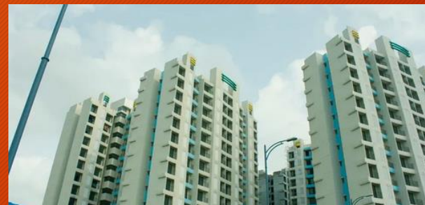
Group Housing Construction
